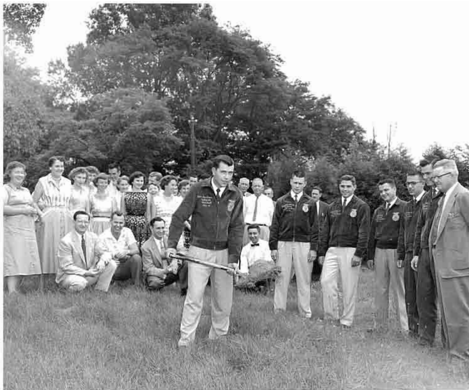
National President Dan Dunham manned the shovel as the 1955-56 National Officer team, FFA Supply Service and The National Future Farmer magazine staffs and National Advisor Dr. W. T. Spanton watched ground being broken for construction of the National FFA Center in Alexandria, Virginia.
