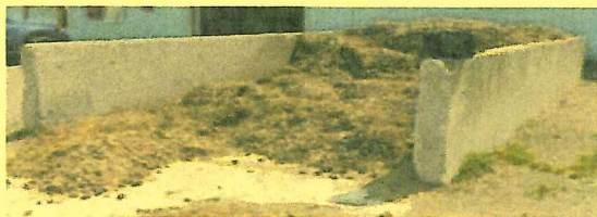
Figure 1: Picture at left is an example of an animal waste storage bay with the floor and three sides constructed from concrete. Stored waste in a bay like this will have additional moisture added by rain and snow and the contaminated runoff is a frequent problem. A new facility is needed to optimized waste handling and storage, and to allow composting of stored waste.
